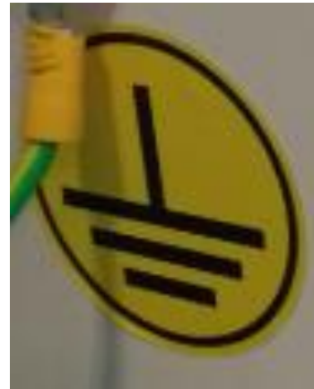
Image :4 Protection Earth
